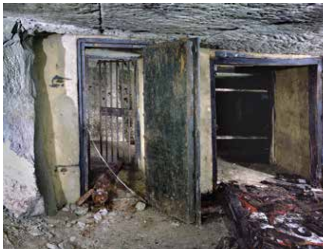
During WWII the western (quarry) part of Marden was cleared of spoil and used as a secure bonded store. The eastern part was used as a hearthstone mine. The internal secure boundary included a subterranean steel door
